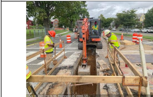
C St NE & 21st St - M8-7 to M8-2 excavation
