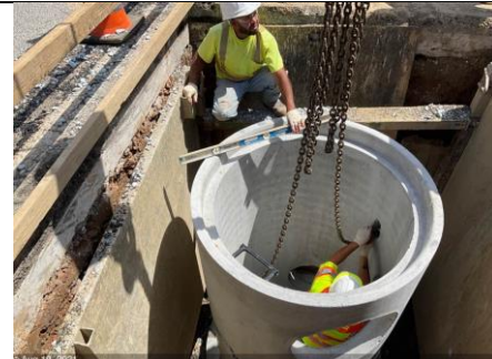
1800 Block C St NE- M6-10 placement
