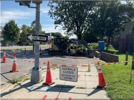
1900 Block C St NE- M7-6 test pit
