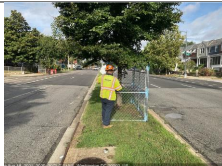
C St NE & 21st St - tree protection installation
