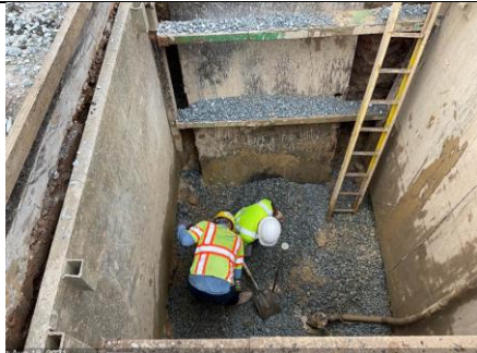
1800 Block C St NE- M6-10 #57 stone placement
