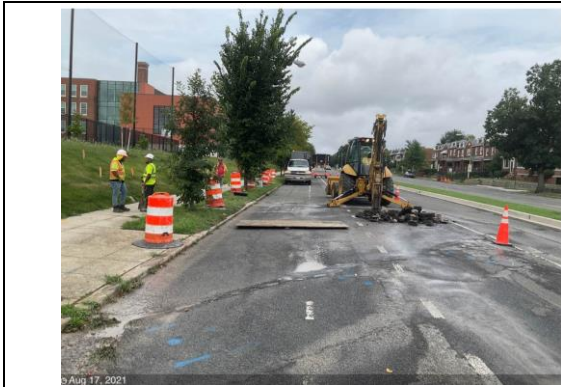
1800 Block C St NE- M6-10 excavation
