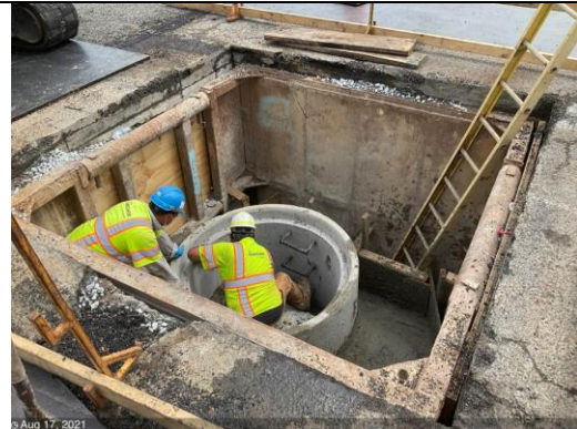
C St NE & 21st St - M8-7 base concrete
