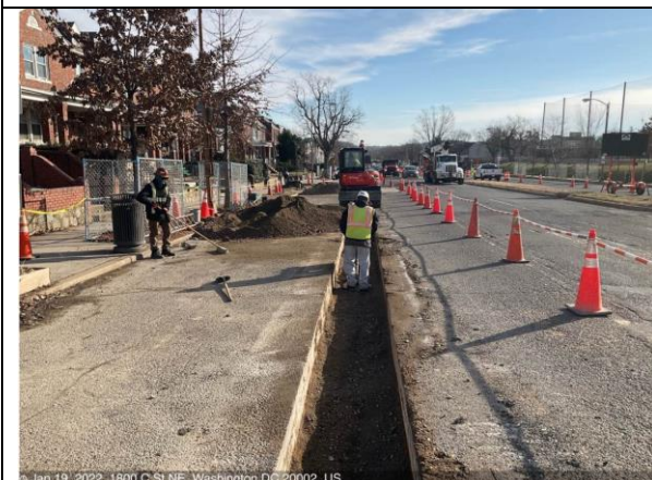
C St NE & 18th PL – Alfaro Backfill between M47 and M49 with RC-6
