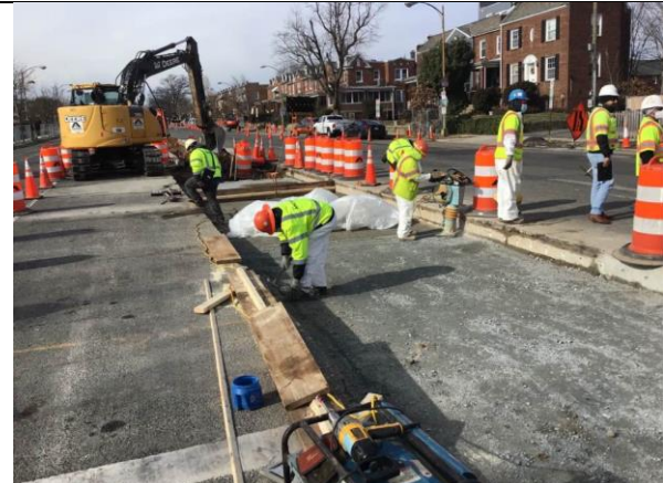
C St NE & 19th – Anchor Prep area for PCC Base
