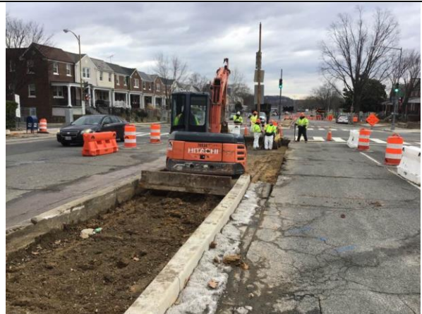
C St NE & 19th – Anchor Excavate and demo median (phase 1F)
