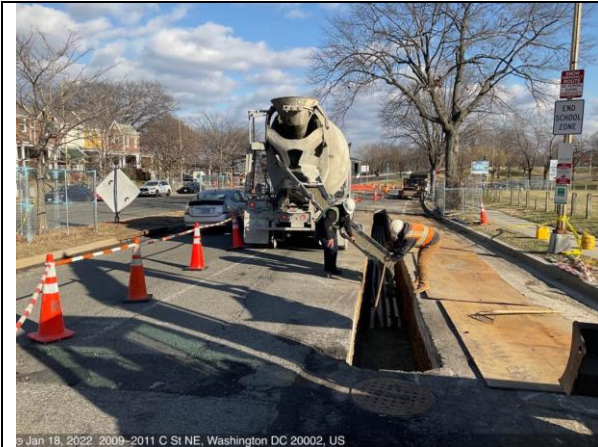
C St NE & 20th – Alfaro Excavate, install conduit, and place concrete between M58 and M61
