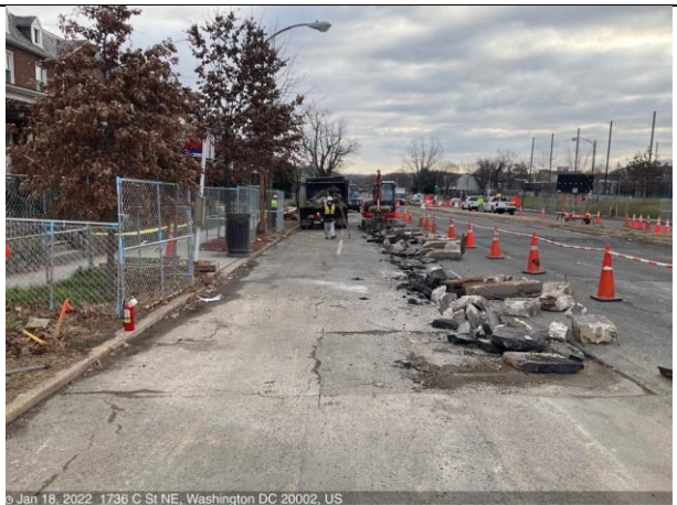
C St NE & 19th – Anchor Excavate and demo median (phase 1F)
