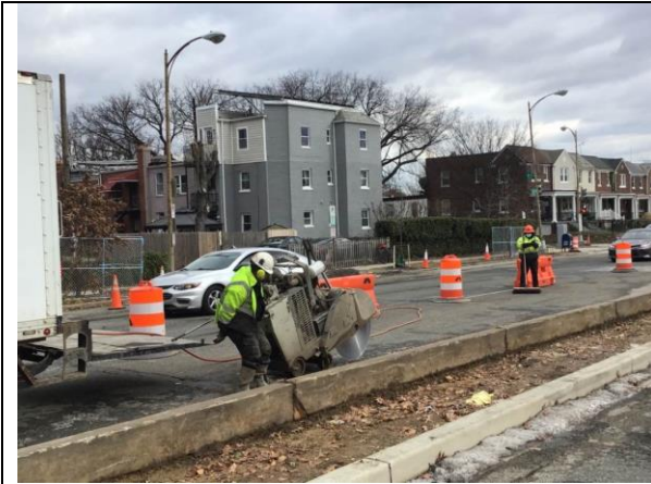
C St NE & 19th – Anchor Sawcut Phase 1F
