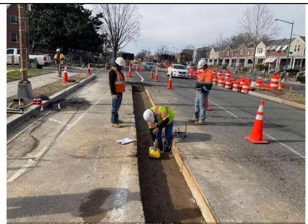
C St NE & 20th – Alfaro Backfill between M58 and M61 with RC-6
