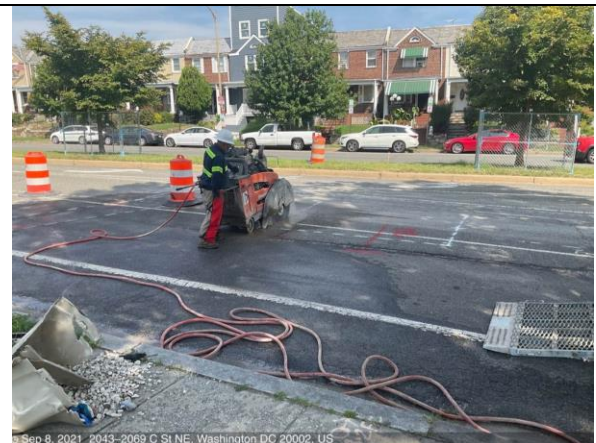
C St NE 2000 Block – Saw cut for M8-2
