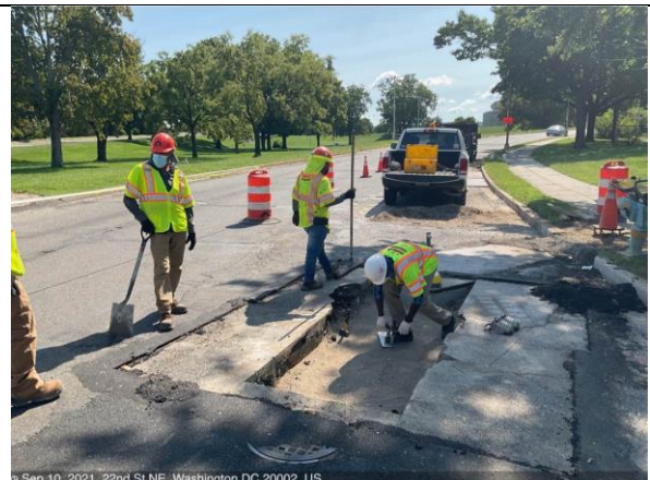
C St NE & 21st St – Backfill 15" RCP between M8-5 to I8-5
