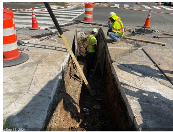
C St NE & 22nd St – Excavate for 15" RCP between M8-1 and I8-1
