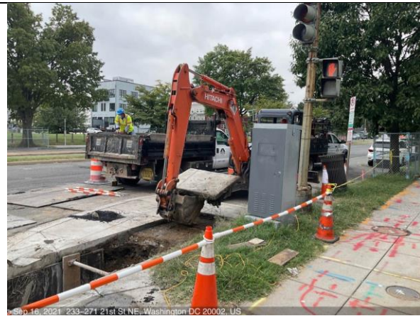
C St NE & 22nd St – Excavate for 15" RCP between M8-1 and I8-1
