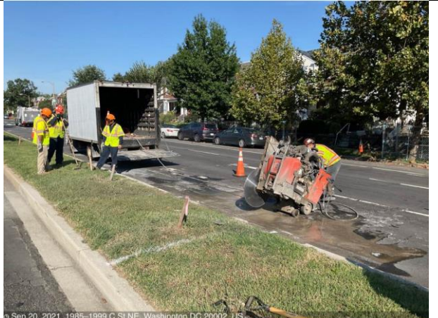
C St NE & 20th – Saw cut and excavate for manhole M7-5
