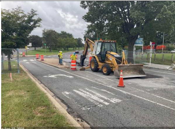
C St NE & 21st – Excavate 15" RCP between M8-7 and M8-2 (RFI 043)
