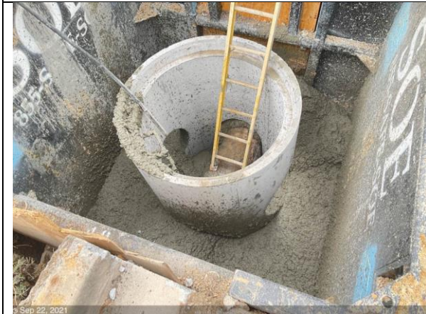
C St NE & 20th – Place concrete for M7-5 base
