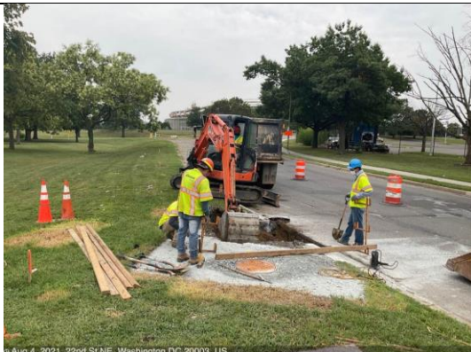
C St NE & 22 nd St – M8-6 to I8-6 excavation
