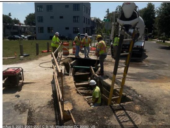
C St NE & 20 th St – M7-4 to I7-12 concrete placement
