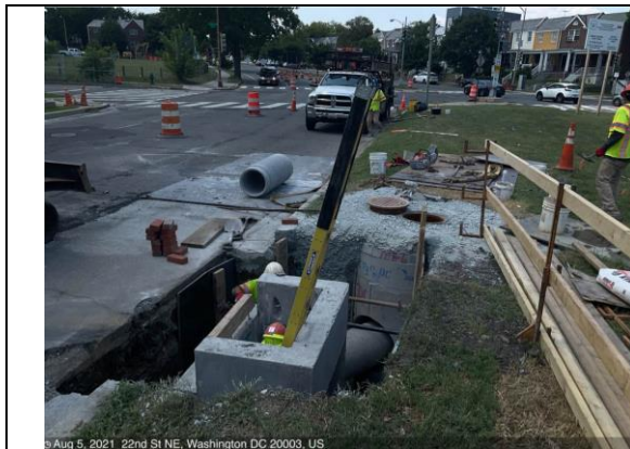
C St NE & 22 nd St – M8-5 to I8-6 RCP placement
