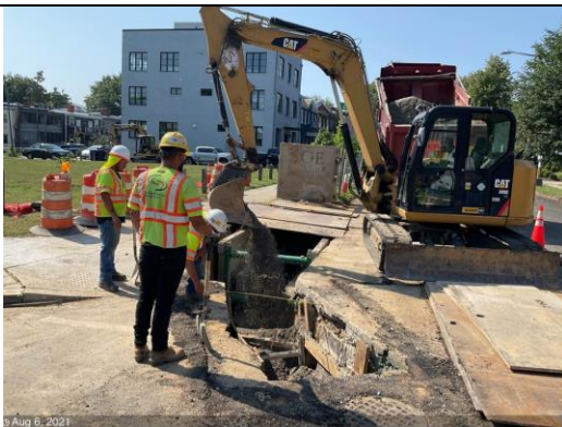
C St NE & 20 th – Backfill of M7-4 to I7-12
