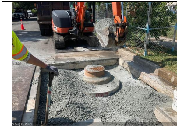
C St NE & 21 st St – M8-4 to M8-3 backfill
