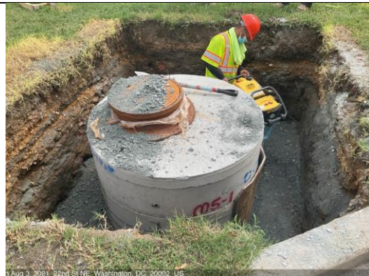
C St NE & 22 nd St – M8-6 backfill
