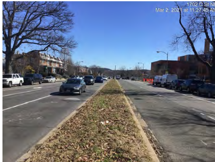
Picture No. 4 – 03022021 – Existing Conditions C St NE at 17 th , looking east
