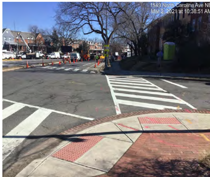
Picture No. 2: 03022021 – WGL Relocation North Carolina at 15th, looking east
