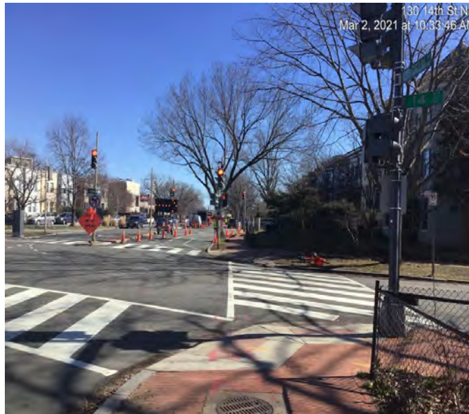
Picture No. 1: 03022021 – WGL Relocation North Carolina at 14th, looking east
