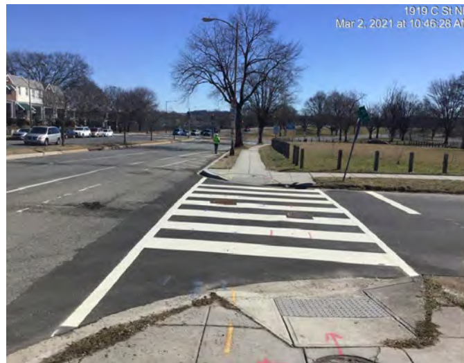
Picture No. 3 – 03022021 – Existing Conditions C St NE at 19th, looking east
