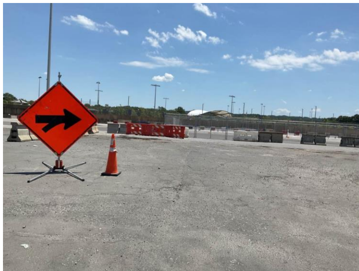
RFK Lot 6 – Lay Down Yard
