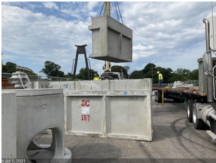
RFK Lot 6 – Drainage Structure Delivery from CP&P
