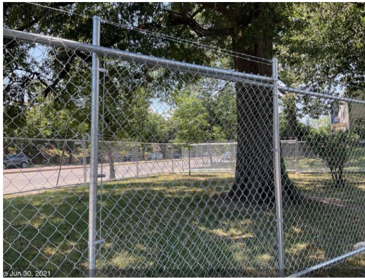
C St NE & 16 th St Park – Repaired Fencing
