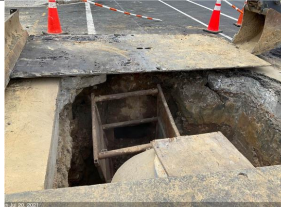
C St NE & 20th St – M7-4 to M7-9 excavation
