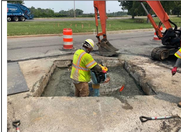
C St NE & 22 nd St – M8-5 CR-6 Backfill
