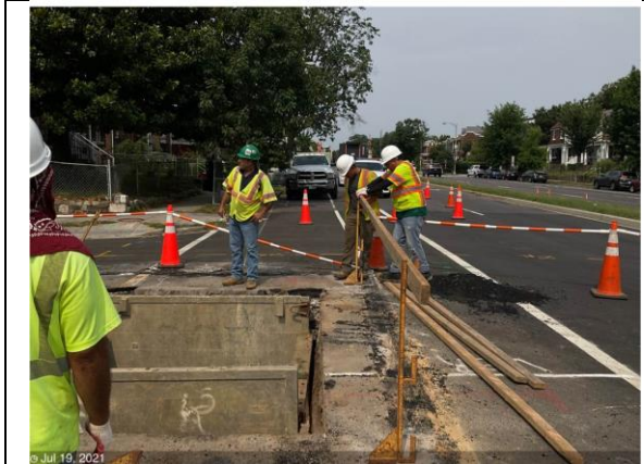
C St NE & 20th St – M7-4 to M7-9 excavation
