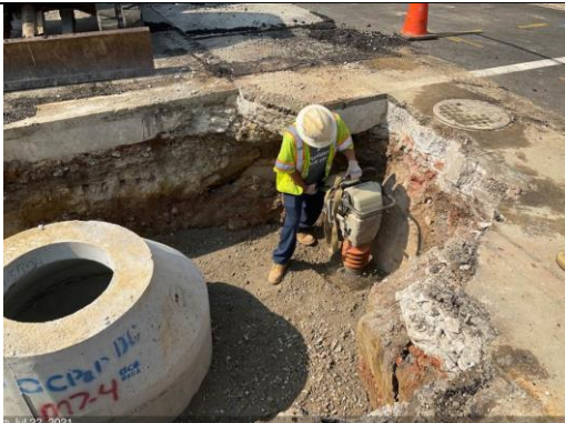
C St NE & 20 th St – M7-4 to M7-9 CR-6 placement
