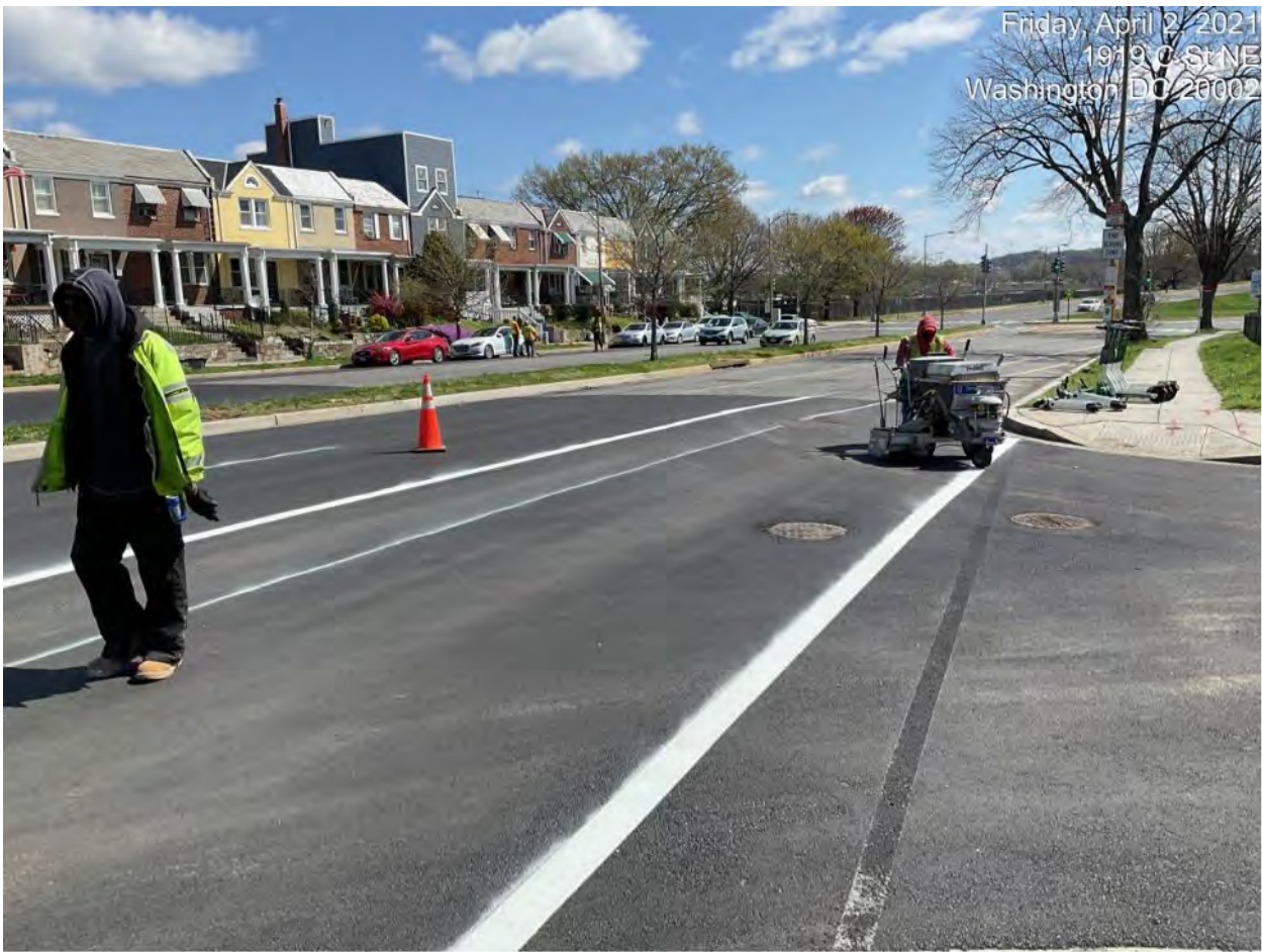
Picture No. 9 – 04022021 – Capital Paving Line Striping C St NE & 20th
