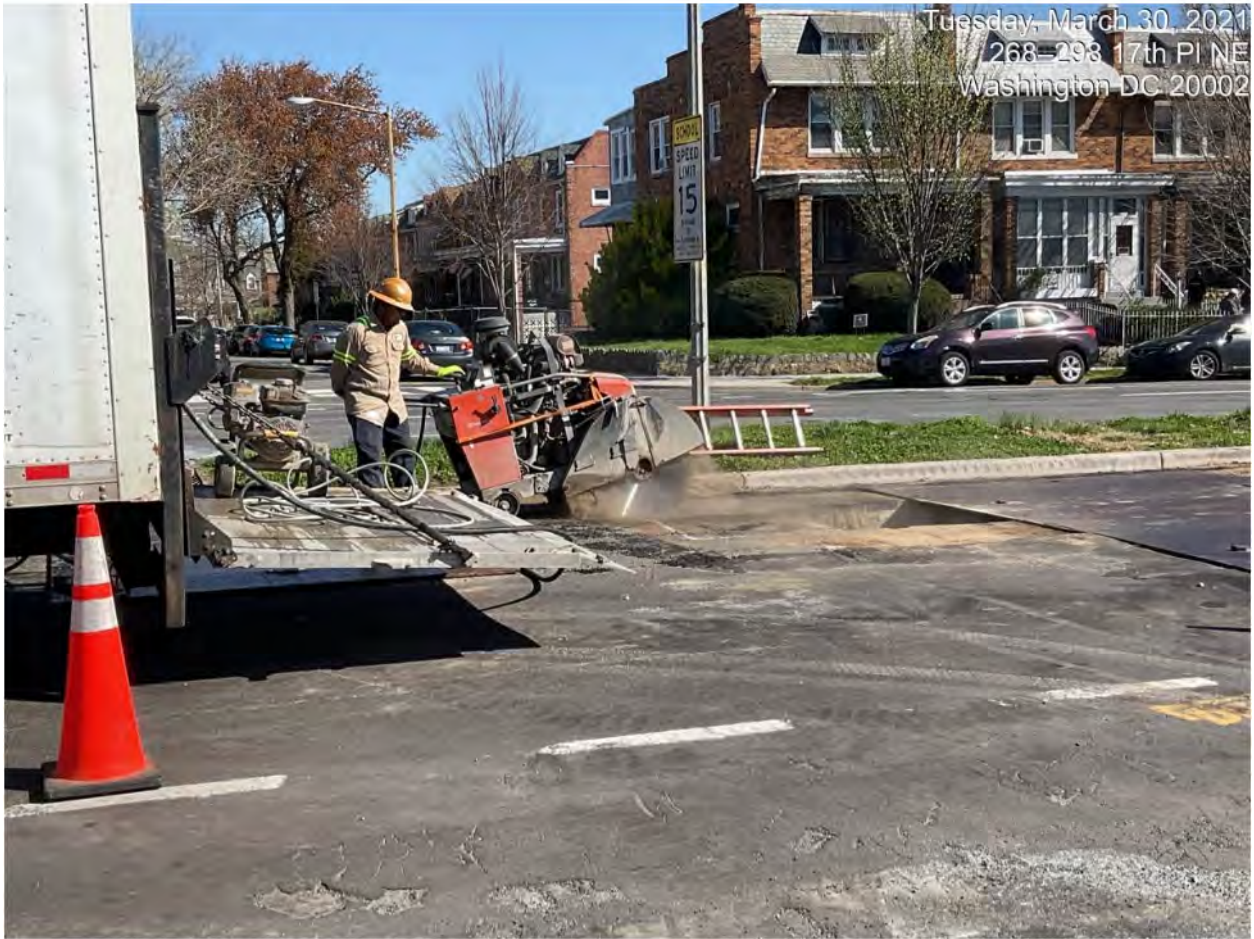
Picture No. 3 – 03302021 – WGL Relocation C St NE & 17th, looking north
