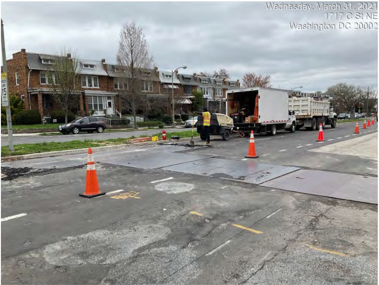
Picture No. 5 – 03312021 – WGL Relocation C St NE & 17th, looking northeast
