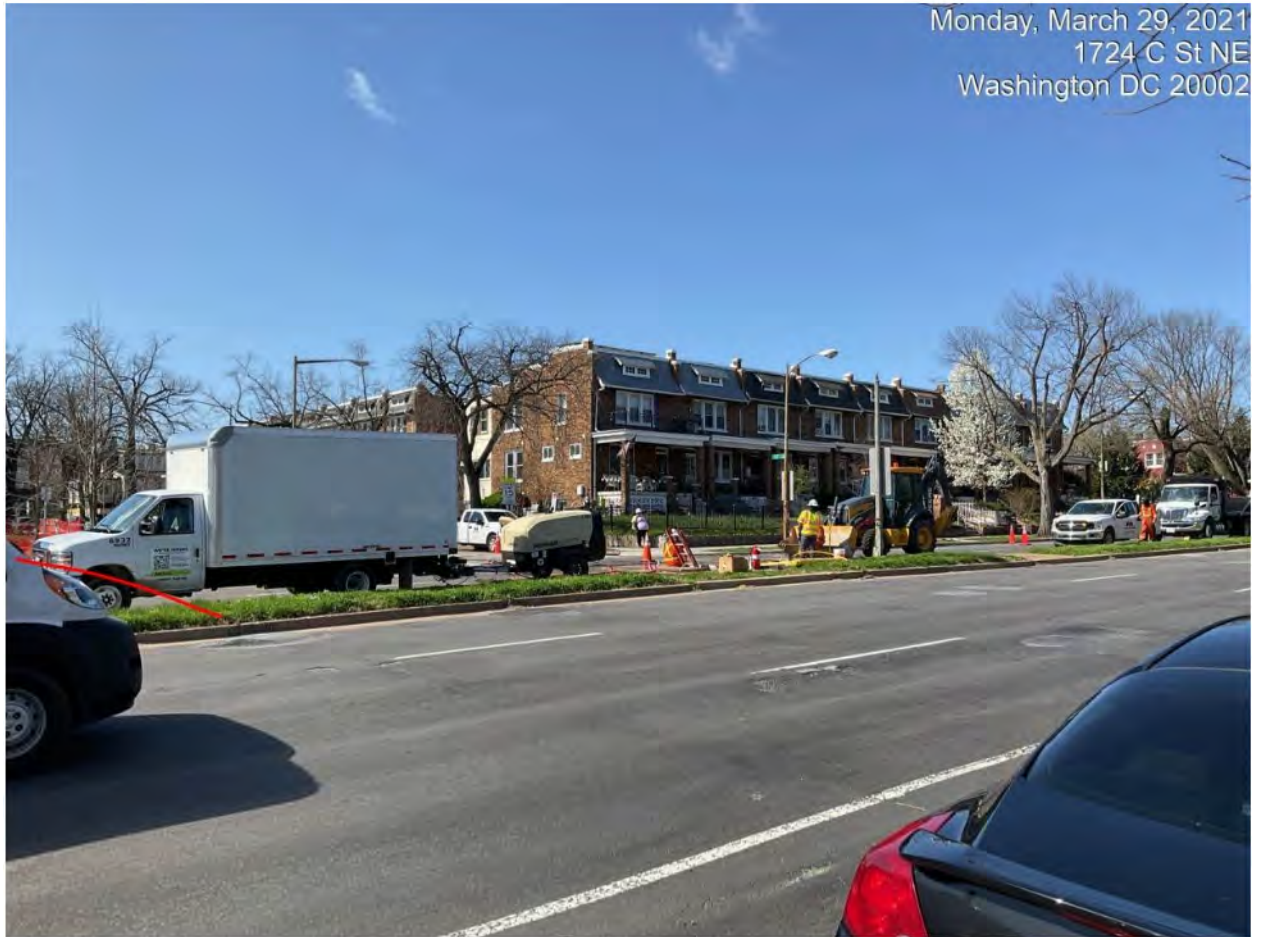
Picture No. 1: 03292021 – WGL relocation, C St NE & 17th looking south
