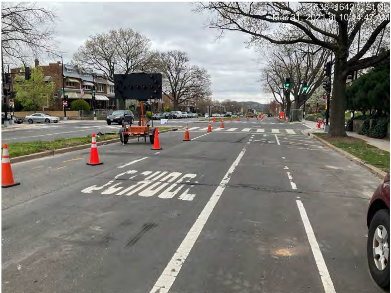
Picture No. 4 – 03312021 – WGL lane closure, C St NE 1600 block, looking east
