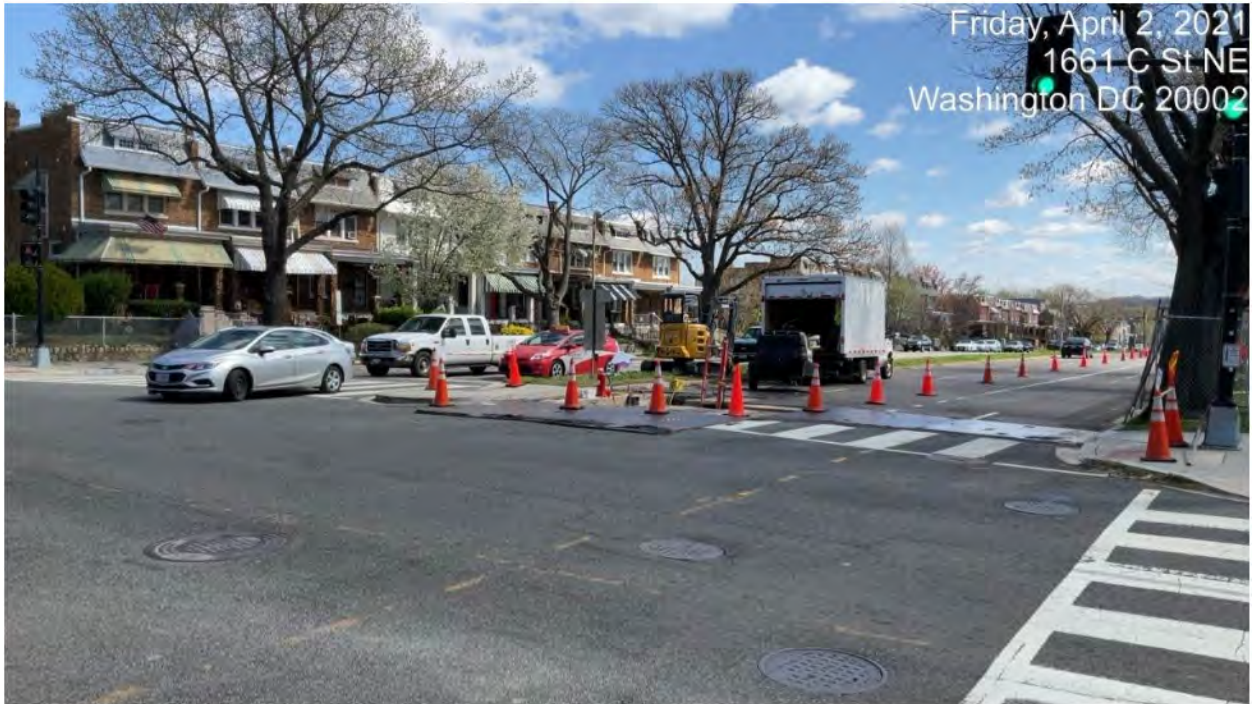
Picture No. 8 – 04022021 – WGL Relocation C St NE & 16th
