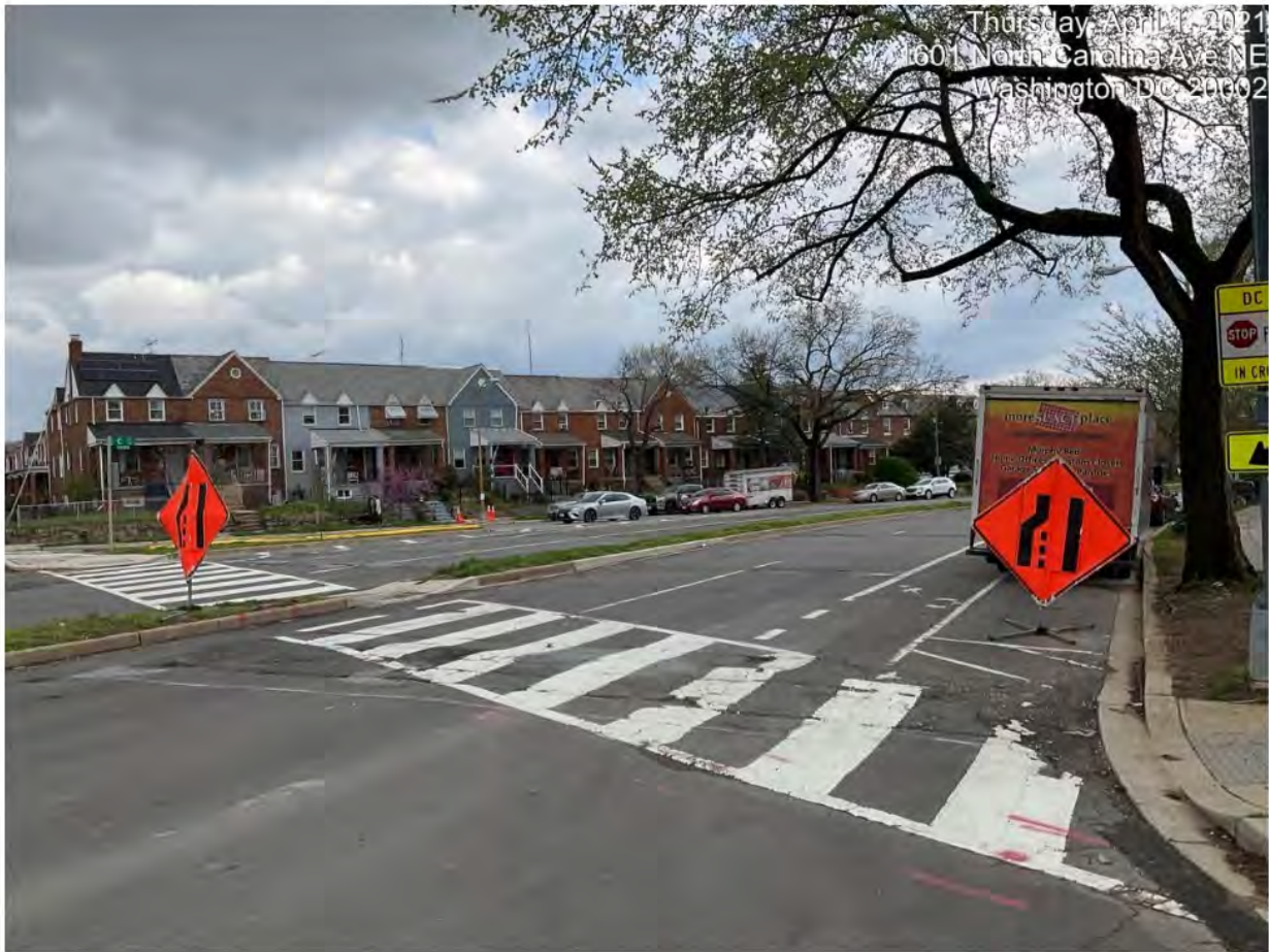
Picture No. 6 – 04012021 – Existing Conditions North Carolina Ave & 16th, looking northeast
