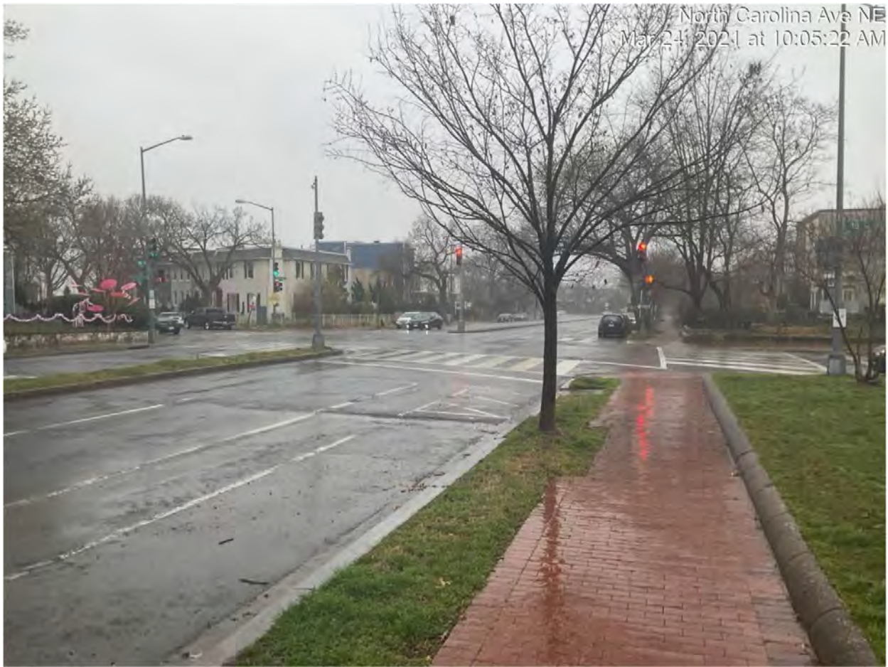
Picture No. 3 – 03242021 – Existing Conditions North Carolina Ave at 15th, looking east
