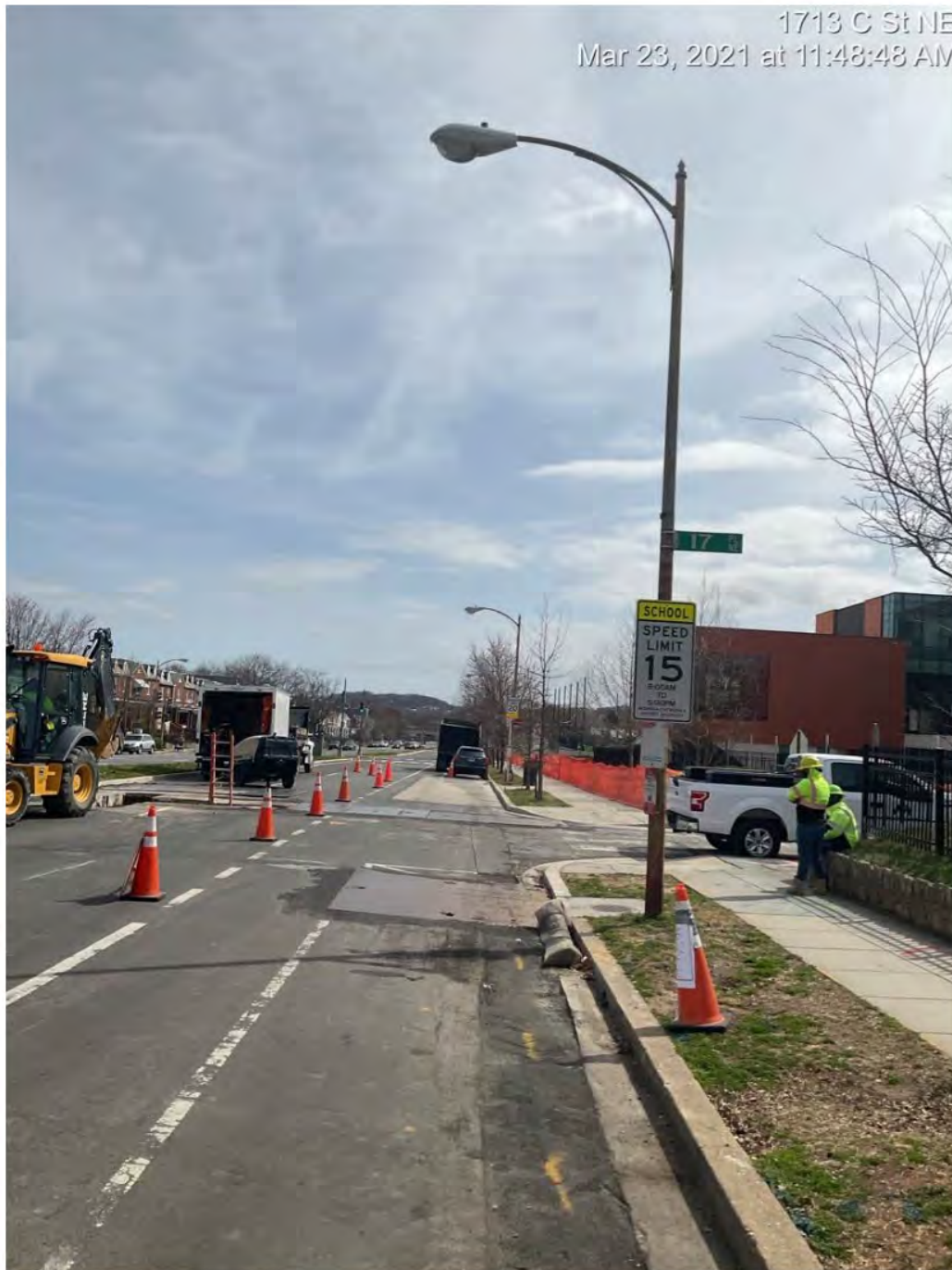
Picture No. 2: 03232021 – WGL Services C St NE at 17th, looking east
