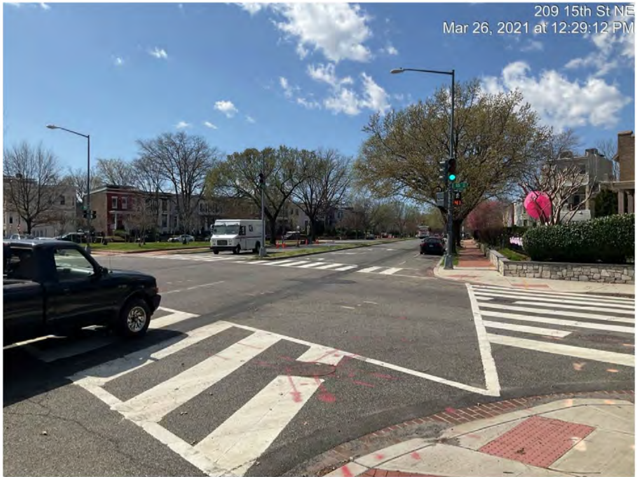
Picture No. 5 – 03262021 – Existing Conditions, North Carolina at 15 th , looking west
