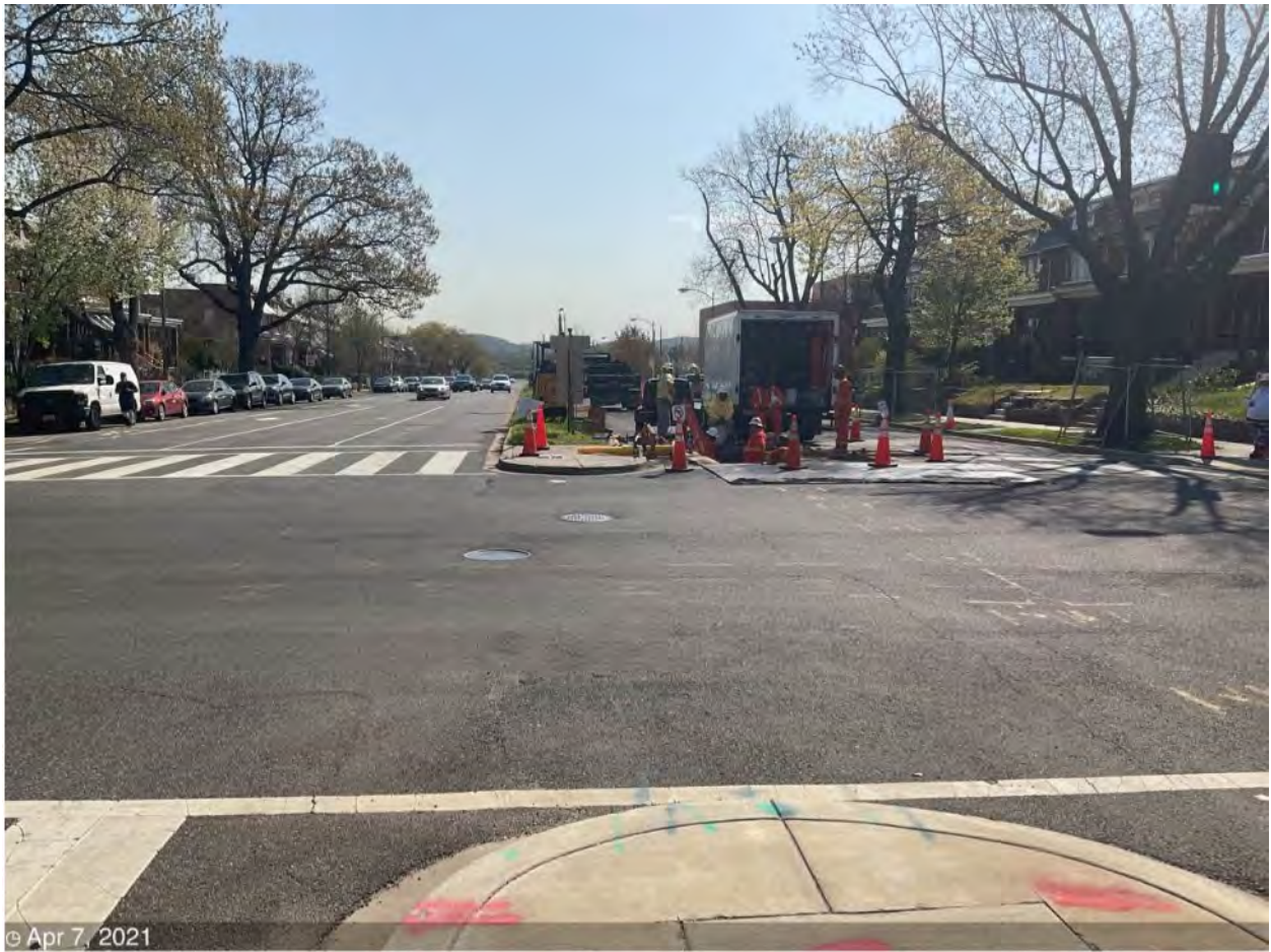
Picture No. 4 – 04072021 – WGL Relocation C St NE & 17th, looking east
