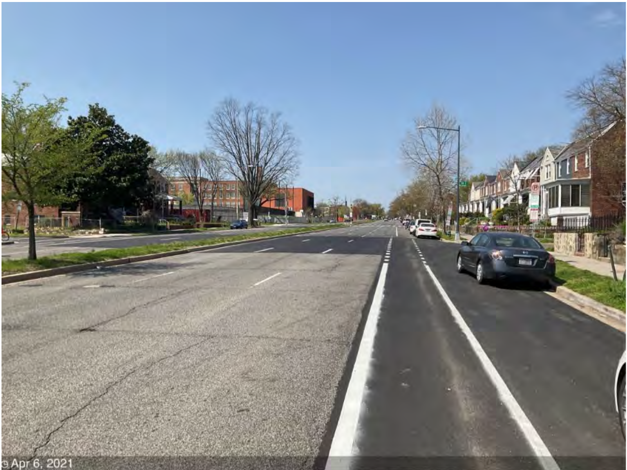
Picture No. 2 – 04062021 – C St NE 2000 block, Verizon roadway restoration, looking west
