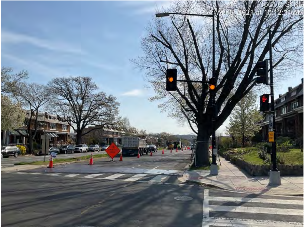
Picture No. 1 – 04052021 – WGL Relocation C St NE & 17th
