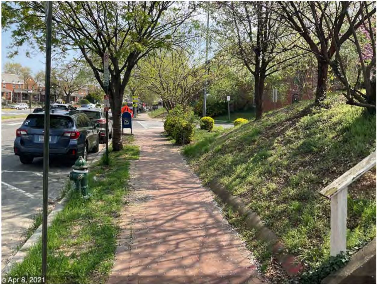
Picture No. 9: 04082021 – Existing Conditions, North Carolina & 16 th looking northeast
