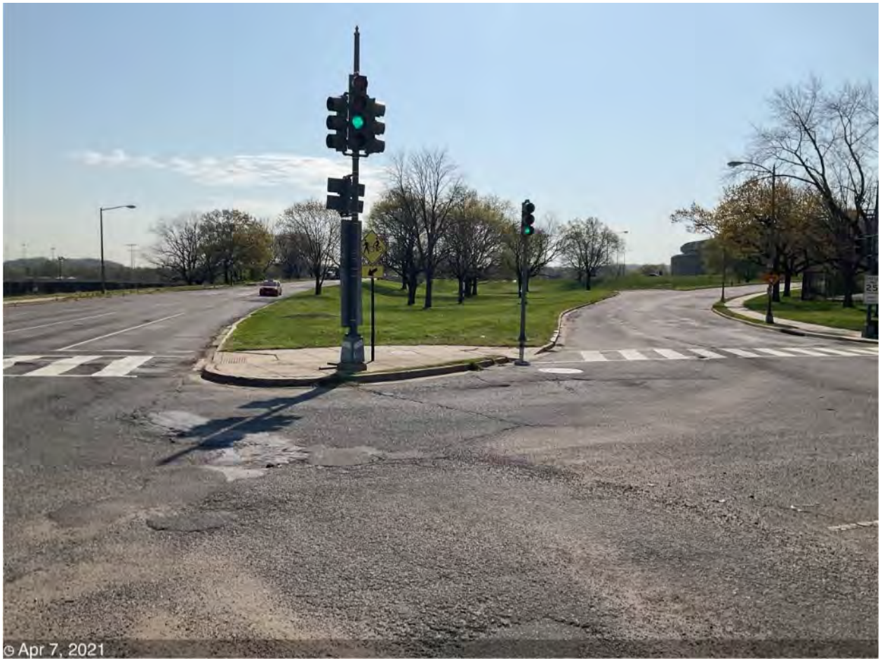
Picture No. 5 – 04072021 – Existing Conditions C St NE & 21st, looking east
