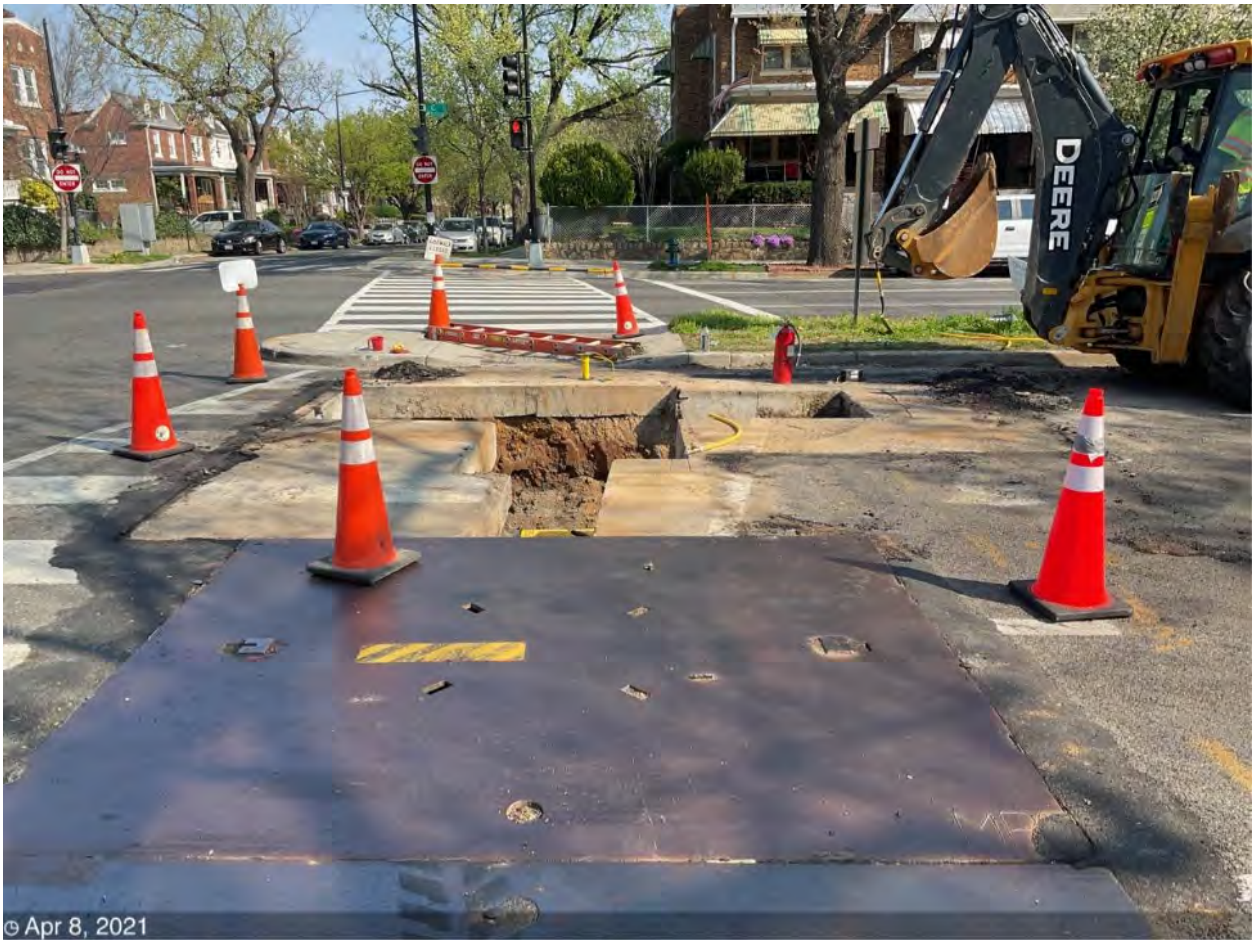
Picture No. 8 – 04082021 – WGL Relocation C St NE & 17th, looking north
