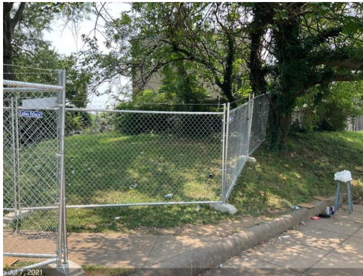
C St NE & 16 th St Park – Fencing
