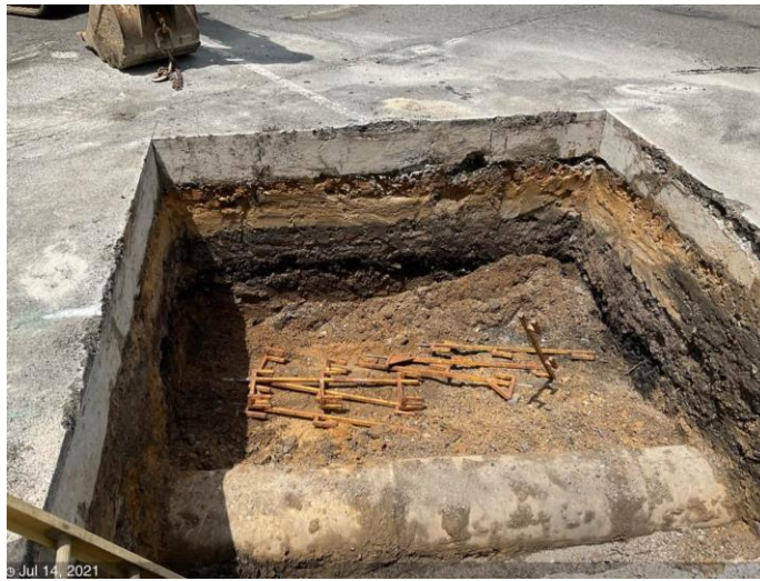
C St NE & 22 nd St – excavate for M8-5
