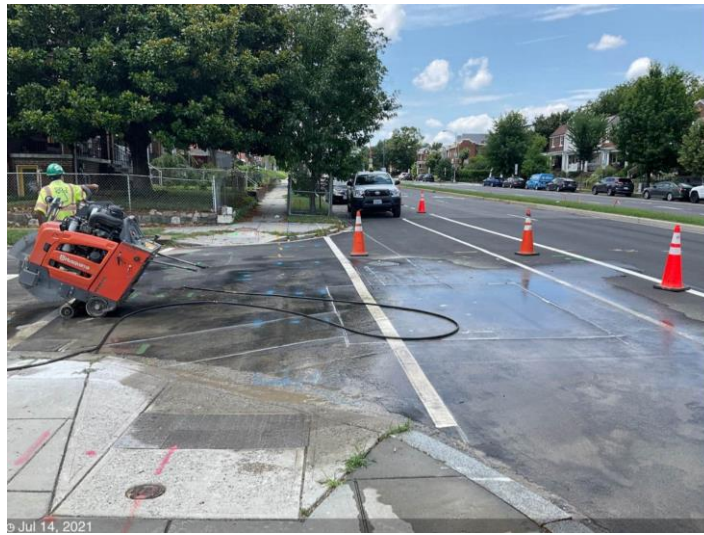
C St NE & 20 th St – saw cut for M7-4
