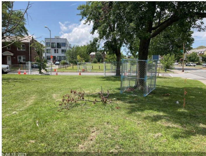
C St NE & 21 st St – Tree Protection Fencing
