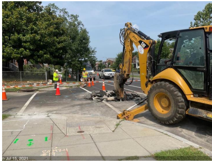
C St NE & 20 th St – excavation for M7-4
